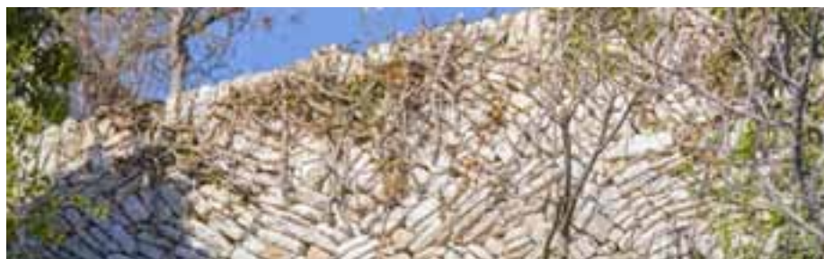
Detail of a dry-stone wall (marogna)
